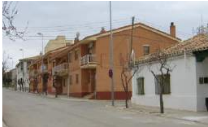
Fachada a C/. Mayor
